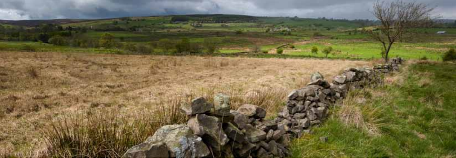
Crumbling walls © PDNPA
