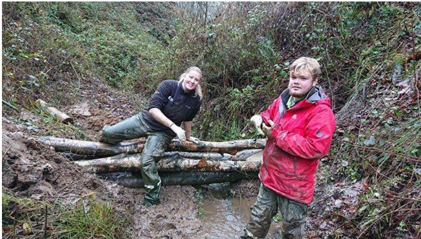
Two apprentices with a dam intended to slow flood water
