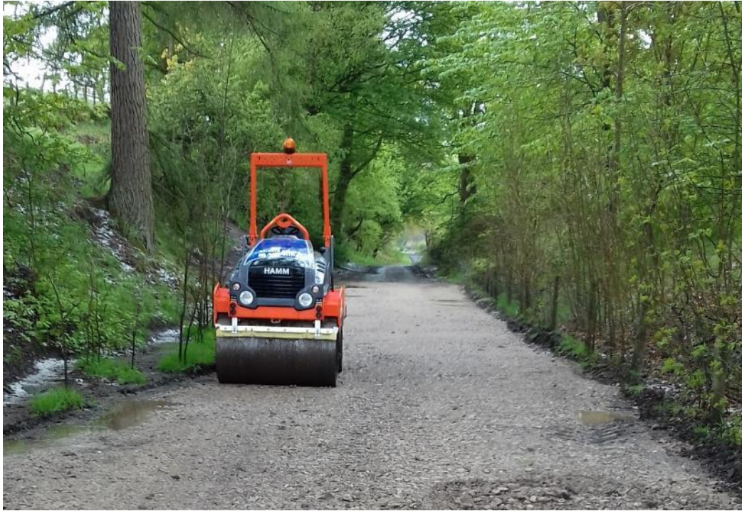
Figure 9. Re-surfacing in progress in May 2019
