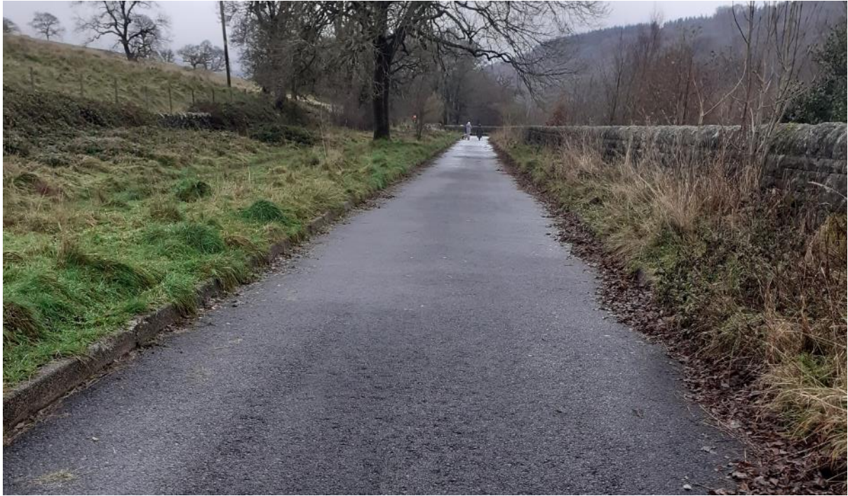
Figure 10. The newly tarmacked approach road
