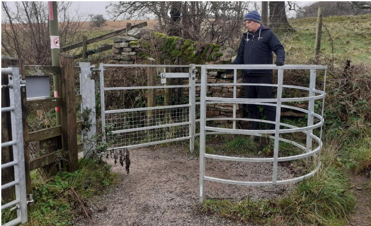
Figure 10. The replacement mobility kissing gates
