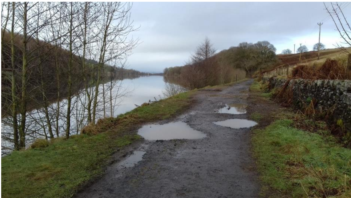
Figure 6. Potholes all along the route
